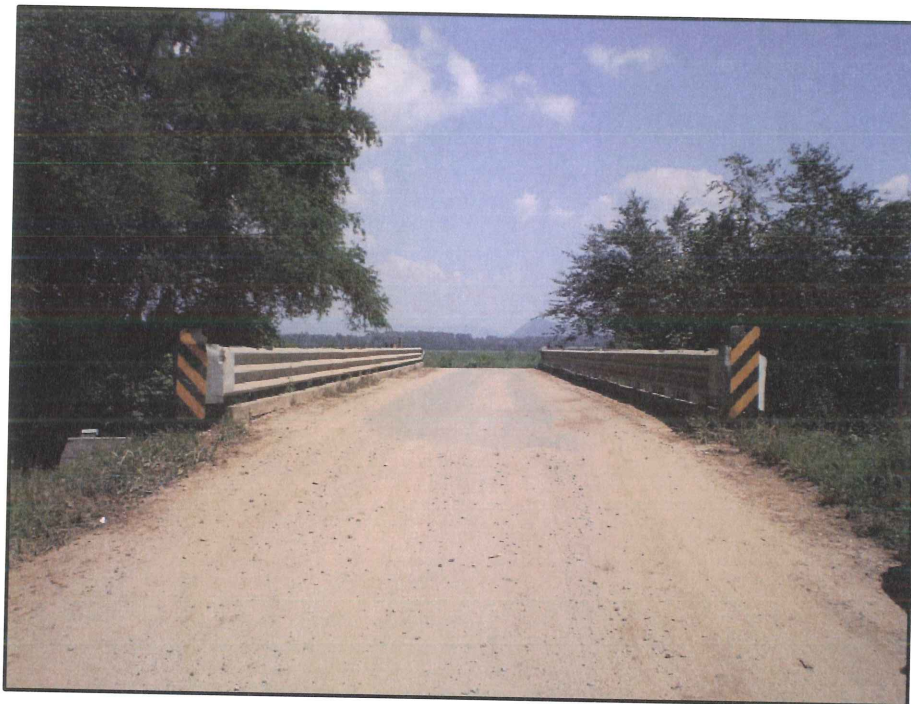
Northbound Approach at bridge
